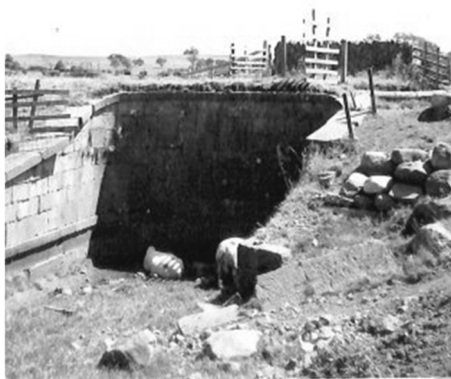
The aqueduct carrying Long Preston Beck over the drainage culvert to the River Ribble, photographed in 1992
